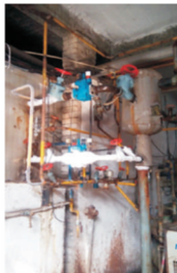
Plant piping after modification
